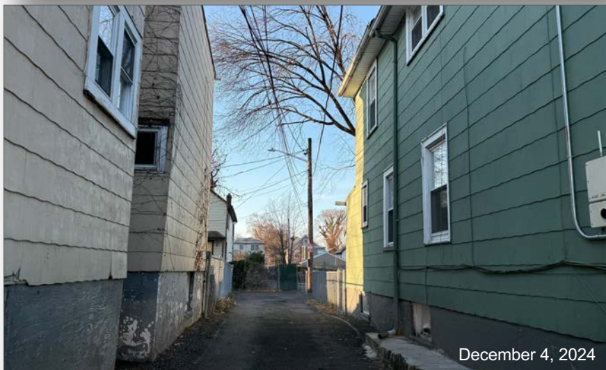
Photo #2: View looking down Berg Place towards the subject property. The Berg Place roadway is 10.3-feet in width.
