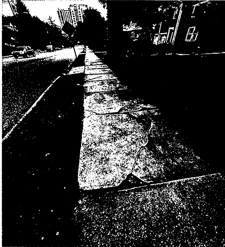
Photo #3 – Damaged sidewalk along Heywood Avenue
