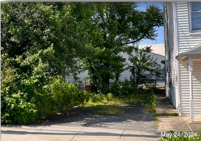
Photo #4: Closer view of the “deed overlap” area. The applicant proposes to attain an access easement from the neighboring property and utilize this area for three (3) parking spaces.
