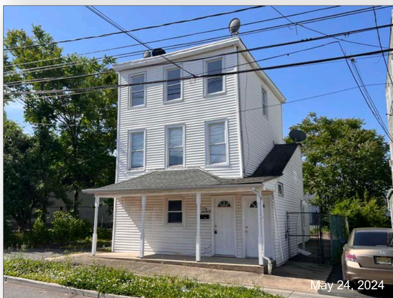
Photo #2: View of the subject property from the west on White Street. Note the two entry doors on the street frontage.
