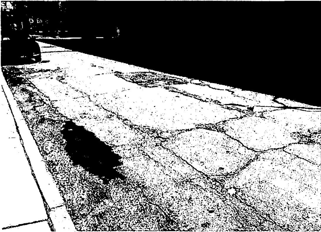
ASPHALT CRACKING
