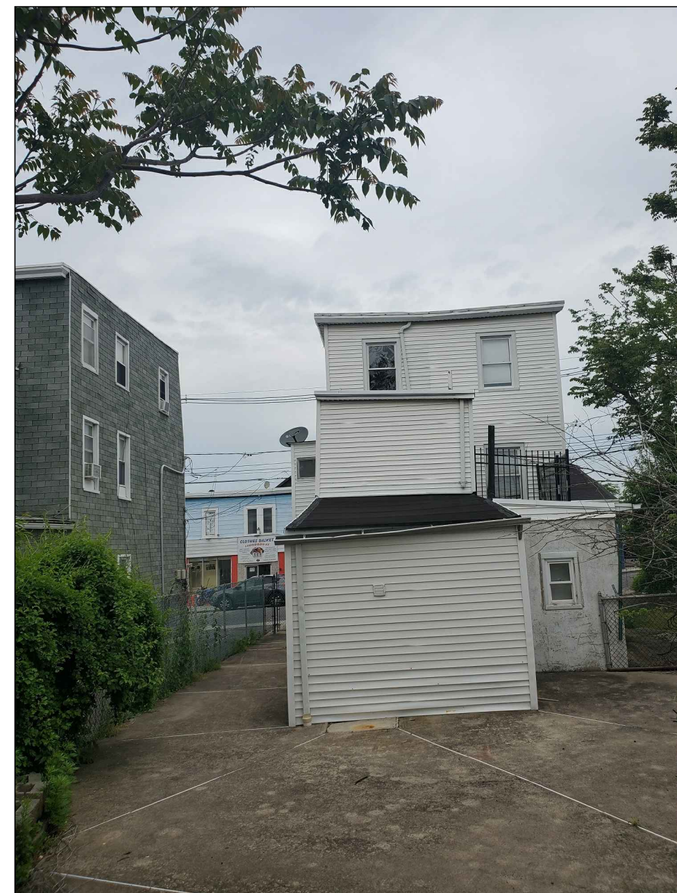
PHOTOGRAPH NO. 4 REAR CENTER VIEW
