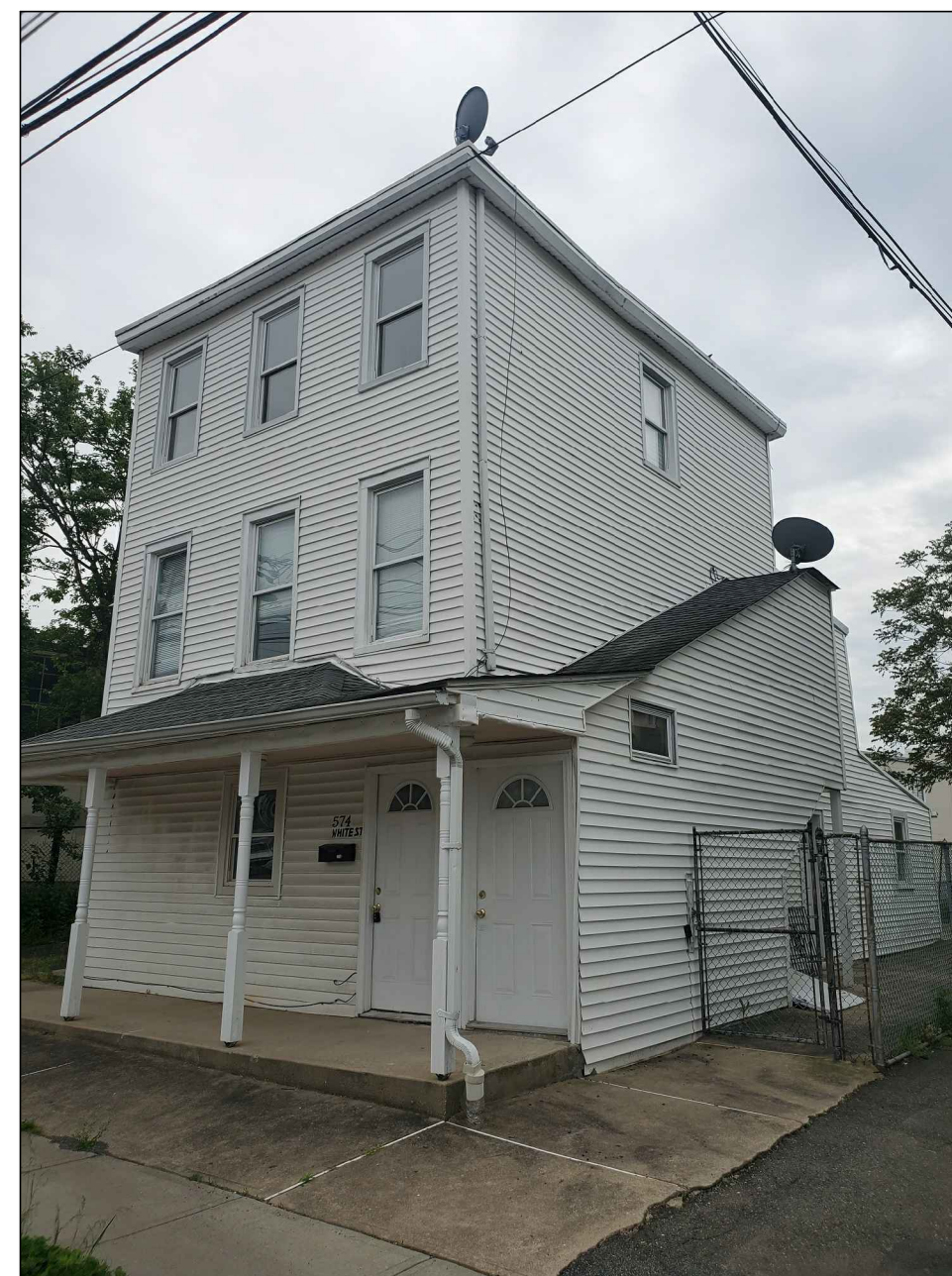
PHOTOGRAPH NO. 3 RIGHT FRONT VIEW
