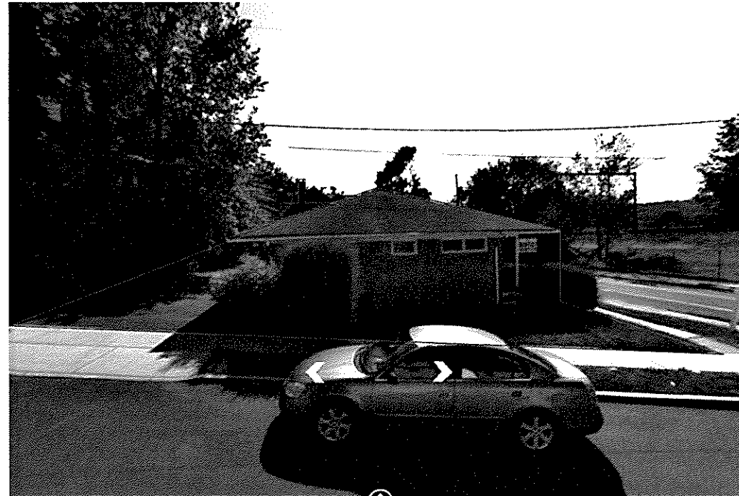
STREET VIEW - HILLSIDE AVENUE
