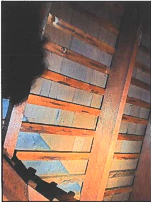
22. Asphalt shingles installed over cedar...
