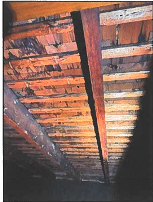
23. Asphalt shingles installed over cedar...
