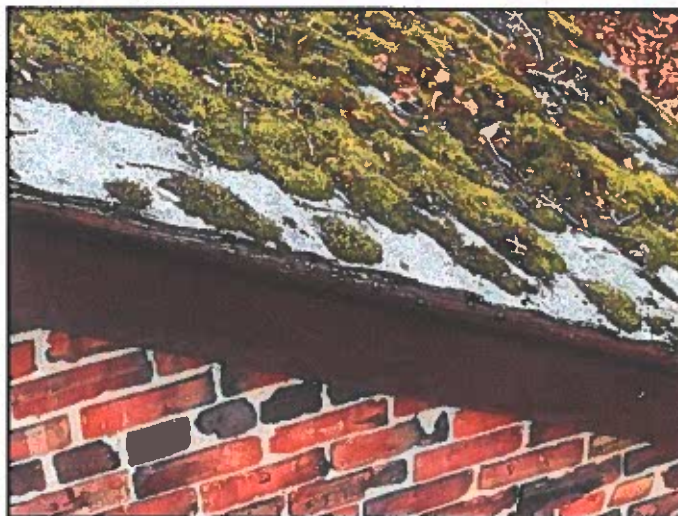
26. Asphalt shingles installed over cedar...
