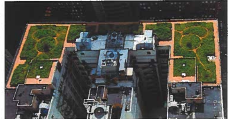
Figure 7: Green Roof Example
