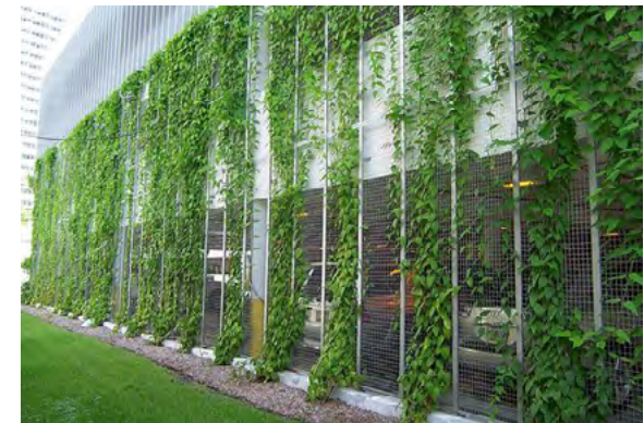
Screening Parking Deck
