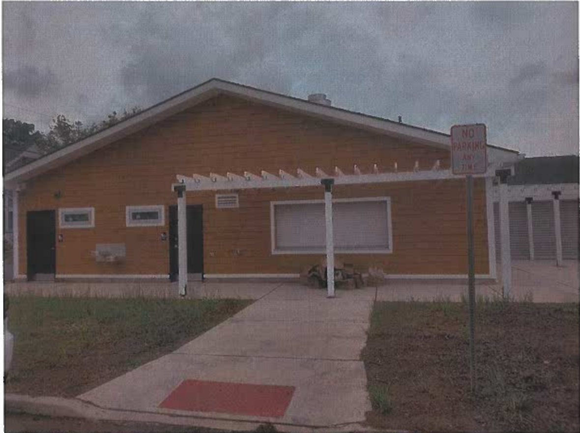
Central Field House (Lincoln Ave Side)
