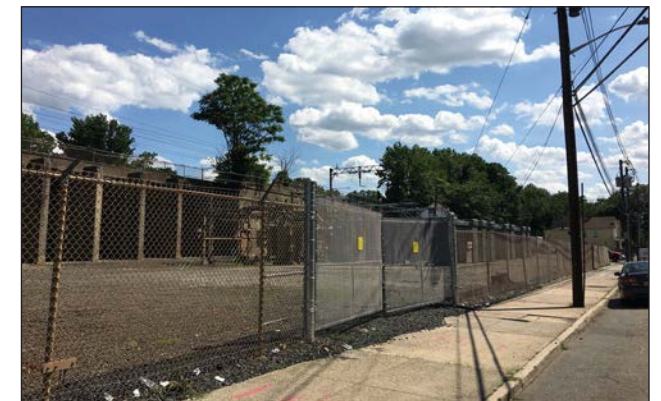
PSE&G Switching Station Site
