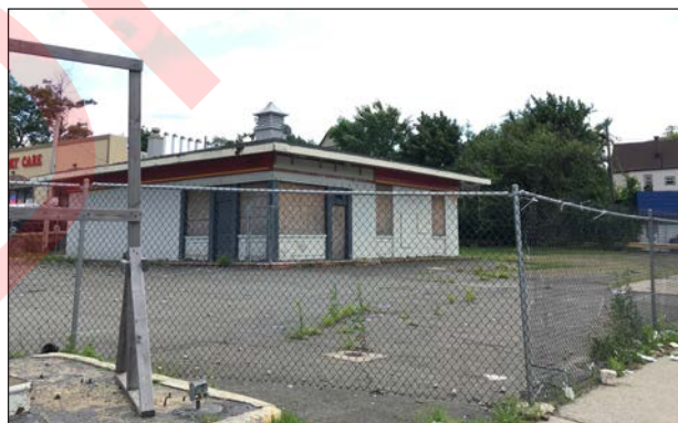
Former Gas Station on corner of Central Ave. and Scotland
