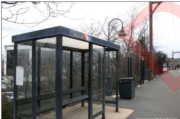
Typical NJ Transit bus shelter
