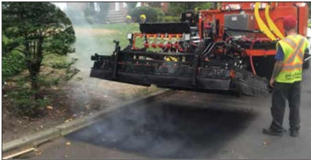
Infrared repair of potholes and pavement trenches
