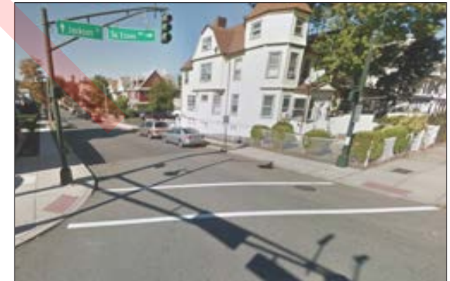
Improvements at Jackson Street showing new curb & ADA Detectable Warning Surfaces
