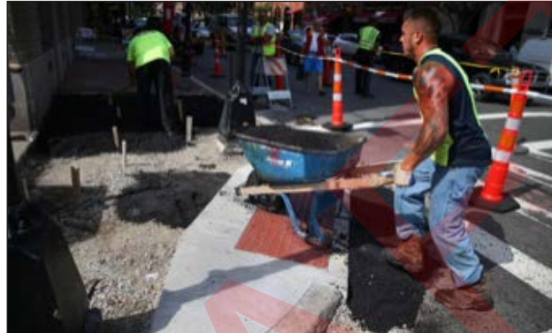
ADA curb ramp and landing under construction (DWS-Detectable Warning Surface shown)
